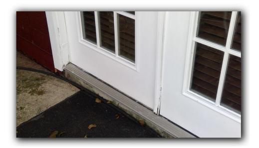
Door frames are out of square and doors have been cut to fit further indicating foundation settlement.
