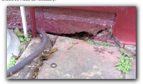
Substantial foundation cracking was observed. This implies that structural movement of the building has occurred. The rate of movement cannot be predicted during a one-time inspection. A structural engineer should be consulted to further evaluate this condition and the remedies available for correction.
