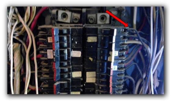
The main distribution panel is crowded with wiring. A larger panel, or an auxiliary panel, would be desirable.
