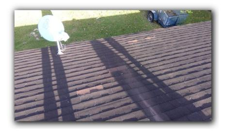
Minor repairs to the roofing are recommended. Damaged or missing roofing material should be repaired. All roof penetrations should be examined and sealed as necessary.
