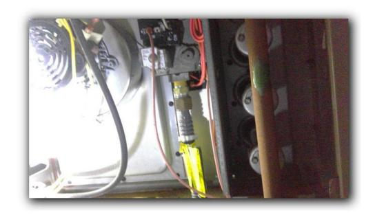
The gas line is not equipped with a sediment trap.
