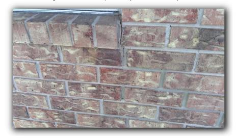
Bowing of the exterior wall structure was observed on the detached garage. This implies that structural movement of the building has occurred. The rate of movement cannot be predicted during a one-time inspection. A structural engineer should be consulted to further evaluate this condition and the remedies available for correction.
