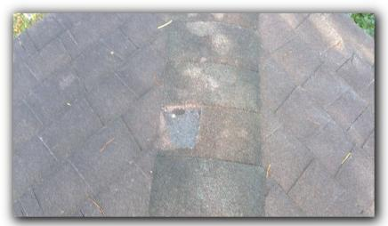
It appears there is more than one layer of roofing shingles installed on the home, but may be covered by felt and a metal drip edge. Further investigation would be needed to verify the number of layers.
