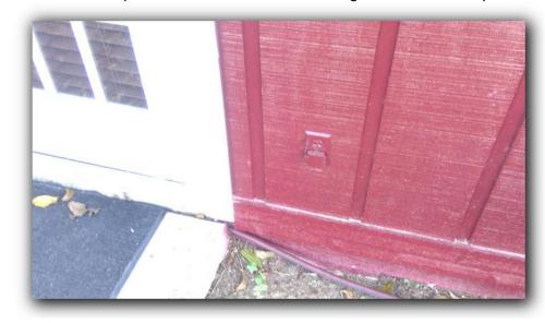
The installation of a ground fault circuit interrupter (GFCI) is recommended in the kitchen, bathrooms, garage, and exterior outlets. A ground fault circuit interrupter (GFCI) offers protection from shock or electrocution.
